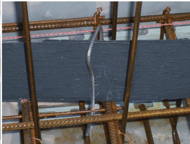
CEMflex VB Plate Waterstop installed prior to the placement of the concrete
