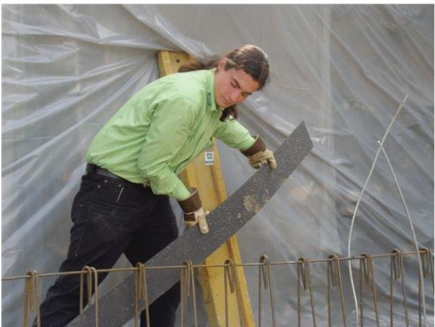
Installation of CEMflex VB Plate Waterstop into the fresh the concrete.
