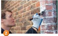
Stormdry can be applied by brush around details such as windows. Care should be taken to ensure that Stormdry does not splash onto glass, paintwork, plants, etc. Any splashes should be cleaned away with warm soapy water.
