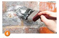
Check for any "missed" areas that have not been treated (e.g. voids in brickwork, deep mortar beds) and apply Stormdry to these areas using a brush.
