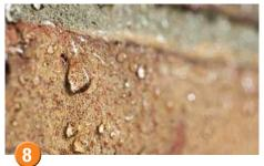
As Stormdry is formulated to penetrate deeply into masonry it can take up to two months after application for a noticeable "beading effect" to appear when rainfall strikes the wall. The masonry will be resistant to light rain after two to four hours.
