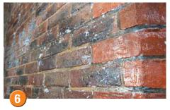
15-20 minutes after application, Stormdry starts to penetrate into the masonry and the whiteness will fade.
